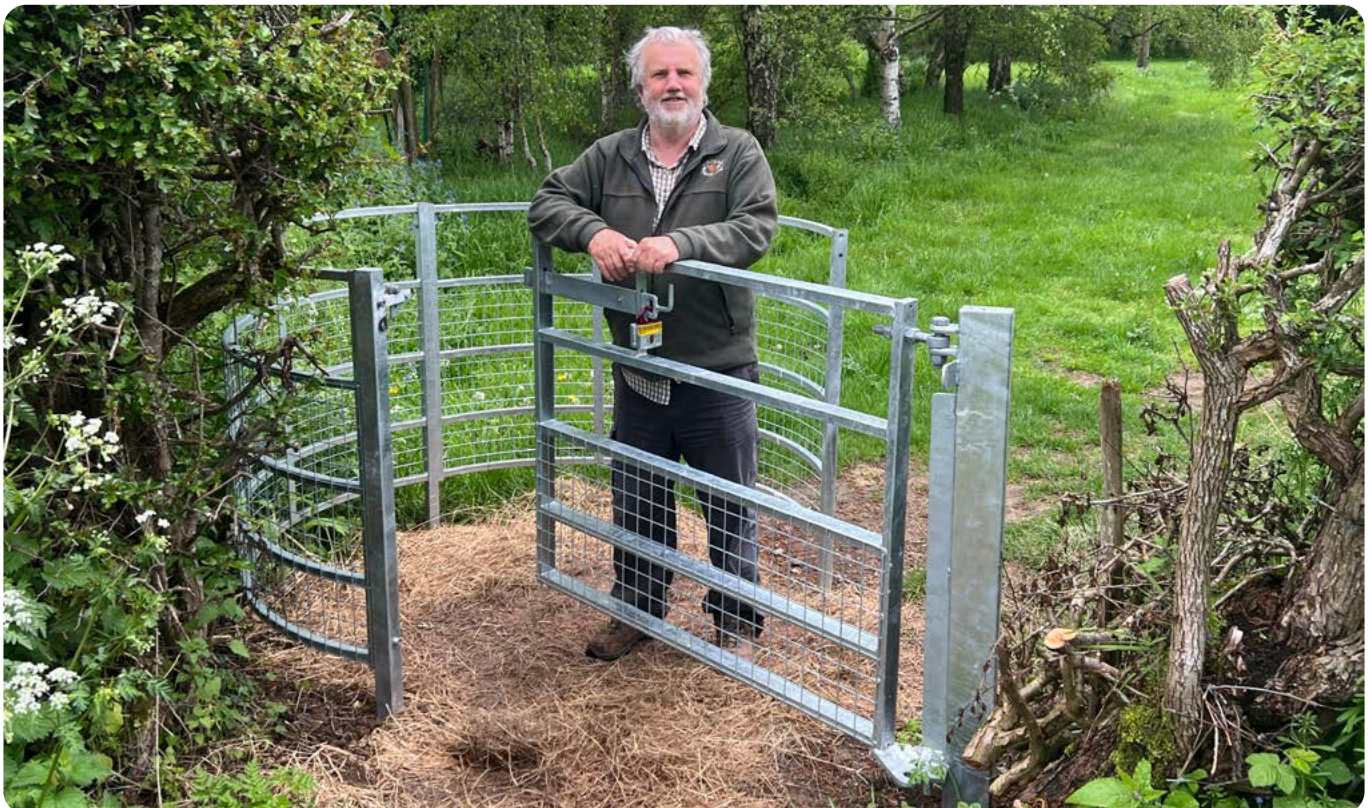
Newly installed access gate, Colwall Village Garden.
