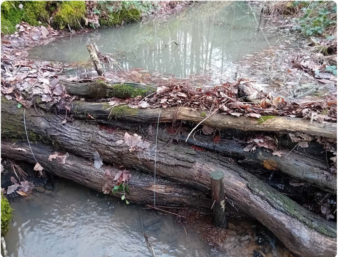
Leaky dam, Worcestershire.
