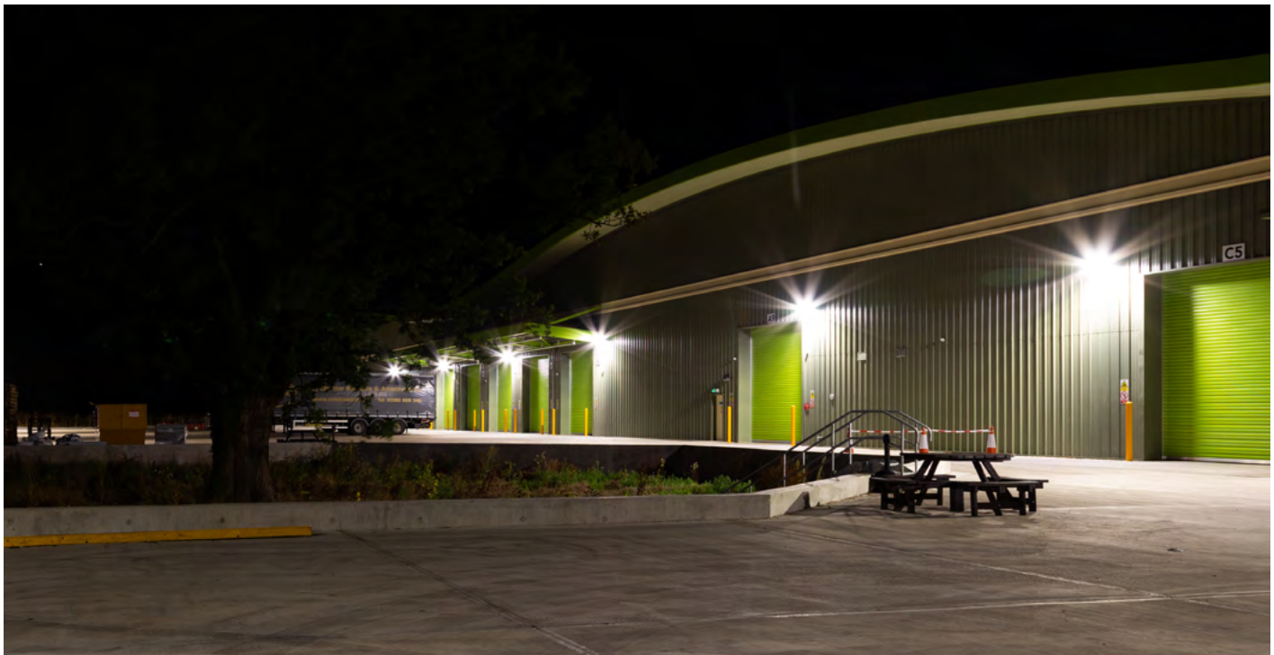
Figure 39 - Downlighters tucked underneath an overhanging canopy close to the building light walkways whilst minimising spill into adjacent areas. This also helps to reduce the effect of night lighting when seen from high ground close by. © Malvern Hills NL Team
