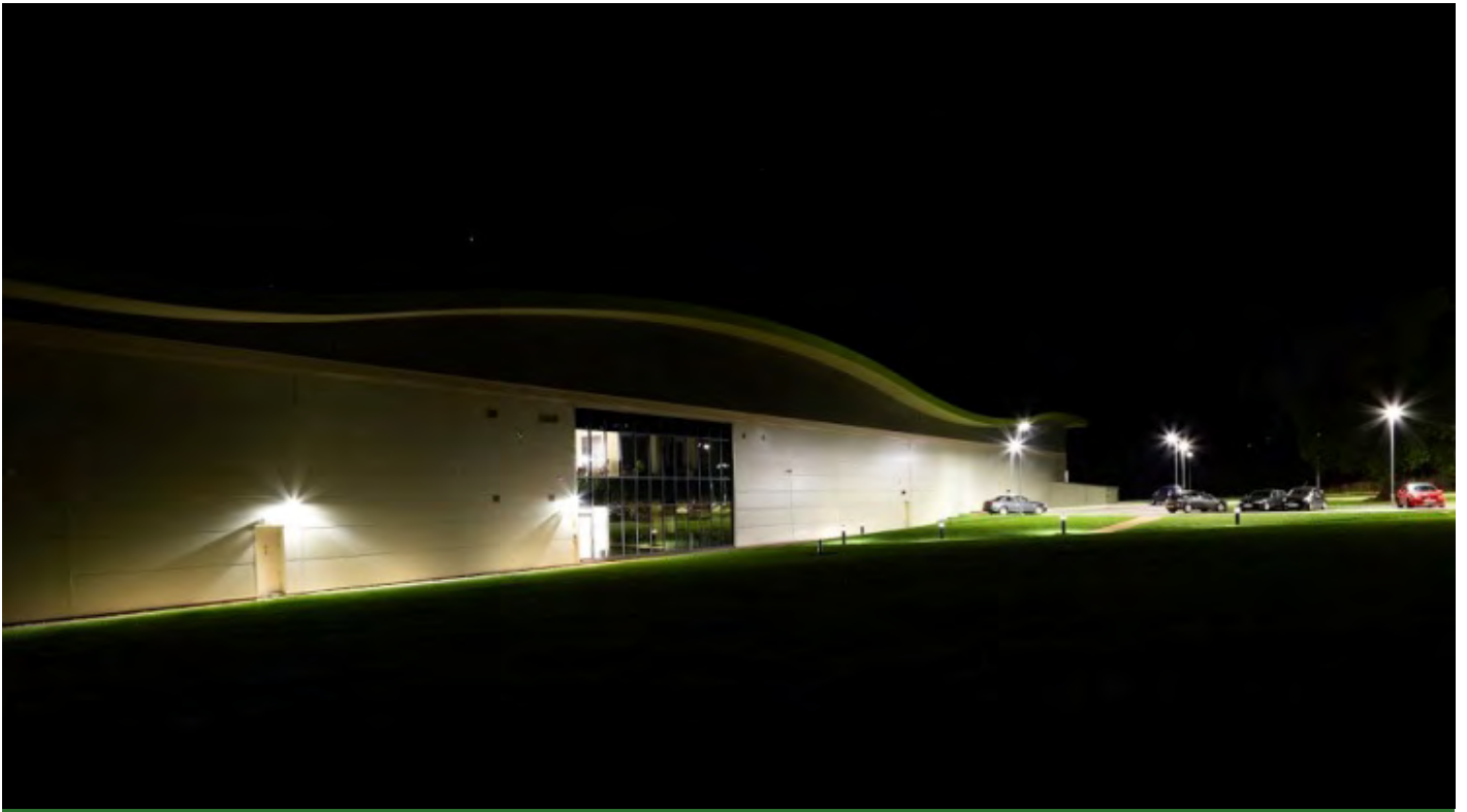
Figure 41 - Restrained site lighting: directional cowls ensure that security lights over main doors have minimum light spillage whilst still providing good lighting levels. High mounted lights in the nearby car park are positioned with luminaires pointing downwards with low beam angles, reducing glare. The spaces between lit areas remain dark.
