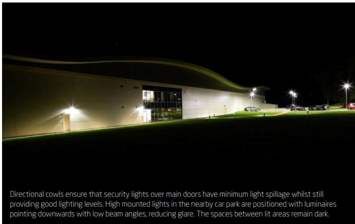
Directional cowls ensure that security lights over main doors have minimum light spillage whilst still providing good lighting levels. High mounted lights in the nearby car park are positioned with luminaires pointing downwards with low beam angles, reducing glare. The spaces between lit areas remain dark.
