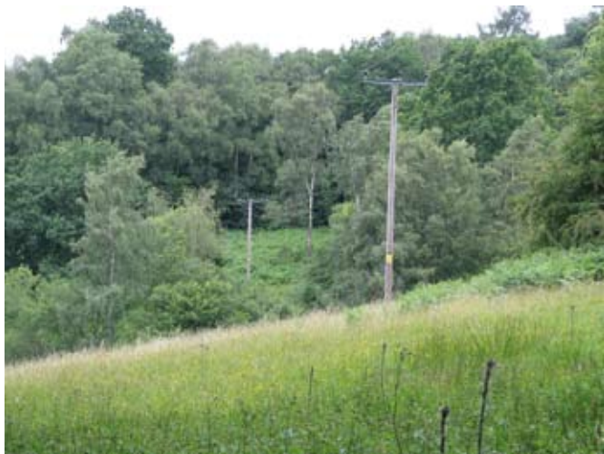
Overhead cables, West Malvern
