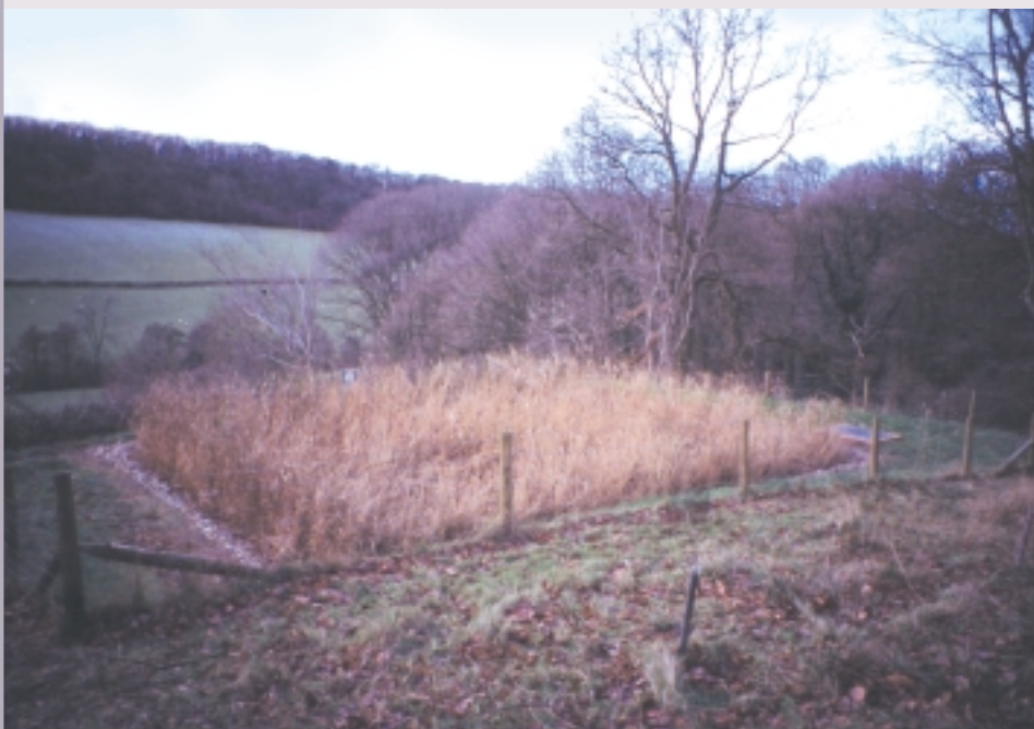
Sewage filtration in a reed bed, West Malvern
