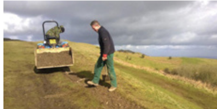
Shire Ditch repairs
