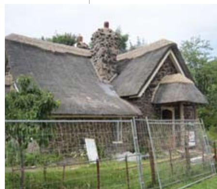
North Lodge after renovation
