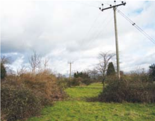
St Wulstan's with overhead lines
