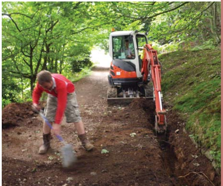
Track restoration works
