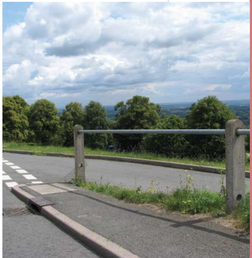
New post and tube fencing
