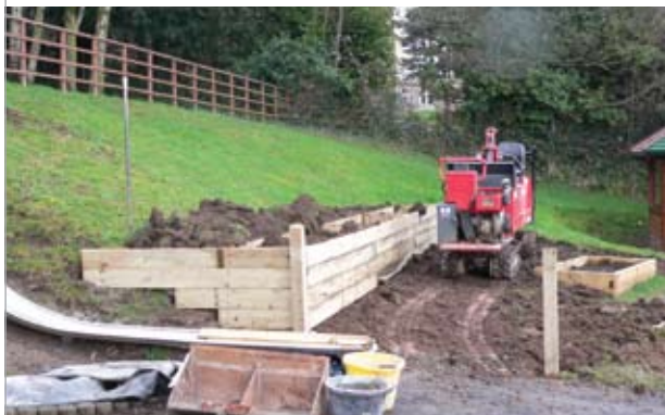
Constructing school eco-garden
