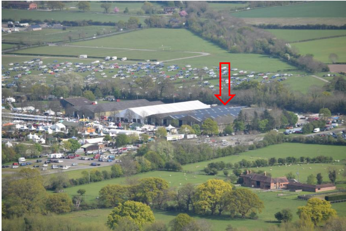
Figure 5.10: New roof cladding on Wye Hall at the Three Counties Showground (AONBLDU10). Colour and finish of new roof material selected to be recessive when seen from the nearby Malvern Hills and not to reflect sunlight.
