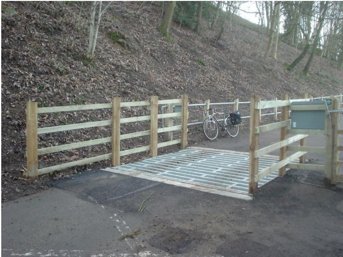
Figure 5.7: Newly installed cattle grid to assist livestock management, British Camp.
