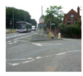
20. Footway alongside road carriageway, from junction with King's End Road, to side turn for field and flood alleviation scheme access. Approximately 290 metres of footway in reasonable condition, variable width, but typically 2.8 metres total width (reduced to 1.8 metres clear width by lamp columns and telegraph poles) along house frontages, and between 1.8 and 2 metres wide beyond the end of the house frontages.
