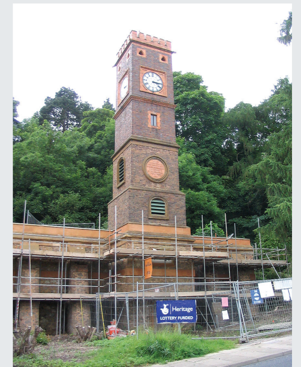
North Malvern Clock Tower - work in progress
