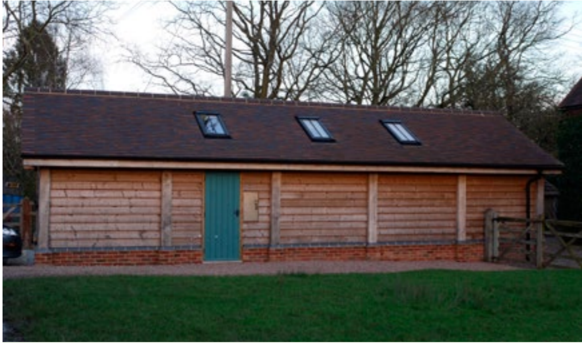
Good colour mix for tiles, timber and brick. In keeping with the Unenclosed Commons Landscape Character Type
