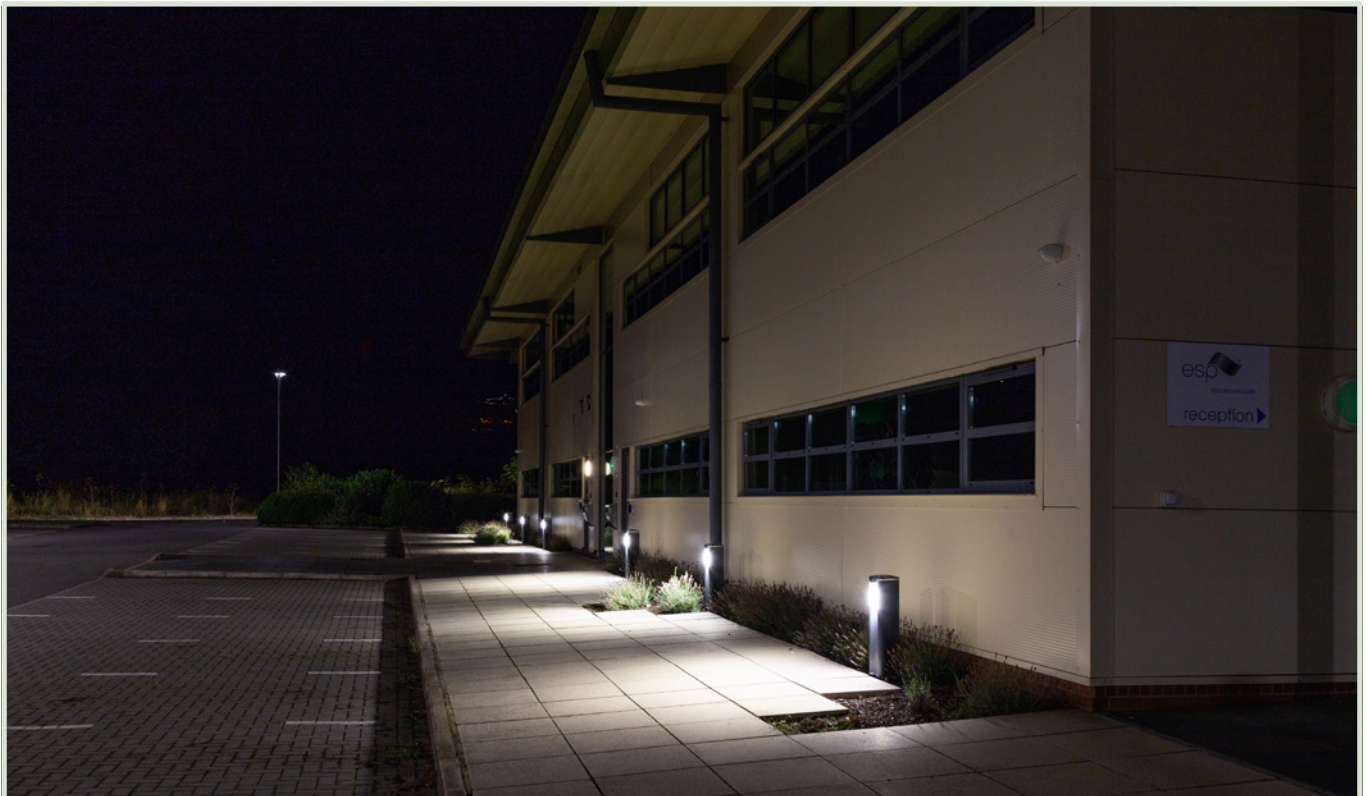
Restrained, well positioned lighting at a warehouse at Blackmore Park, Malvern
