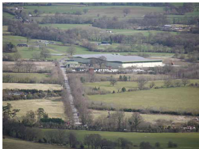
Figure 4 A building too large for its setting and in conflict with the alignment of the prominent avenue
