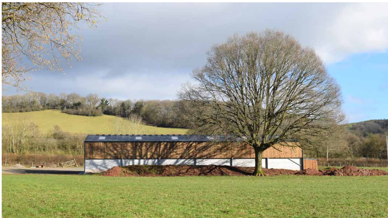
Figure 21 Mature tree in front of a new barn
