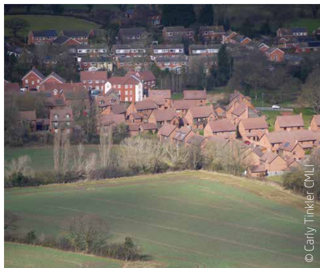
Figure 19 Dense housing rendered less visible through good selection of colour and material including the absence of white trim; where white has been applied, it is highly conspicuous
