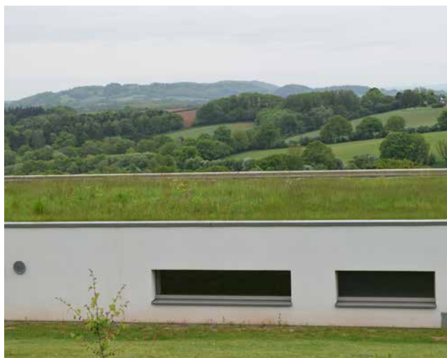
Figure 17 Green roof integrates built form successfully into views of surrounding landscape, but contrasting white elevation and trim draw the eye
