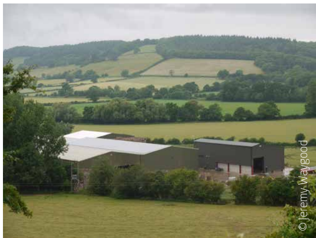
Figure 14A Light-coloured roofs draw the eye and disrupt the view more than those which are darker
