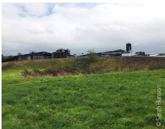
Figure 10 Cut and fill used to create a flat platform on sloping ground
