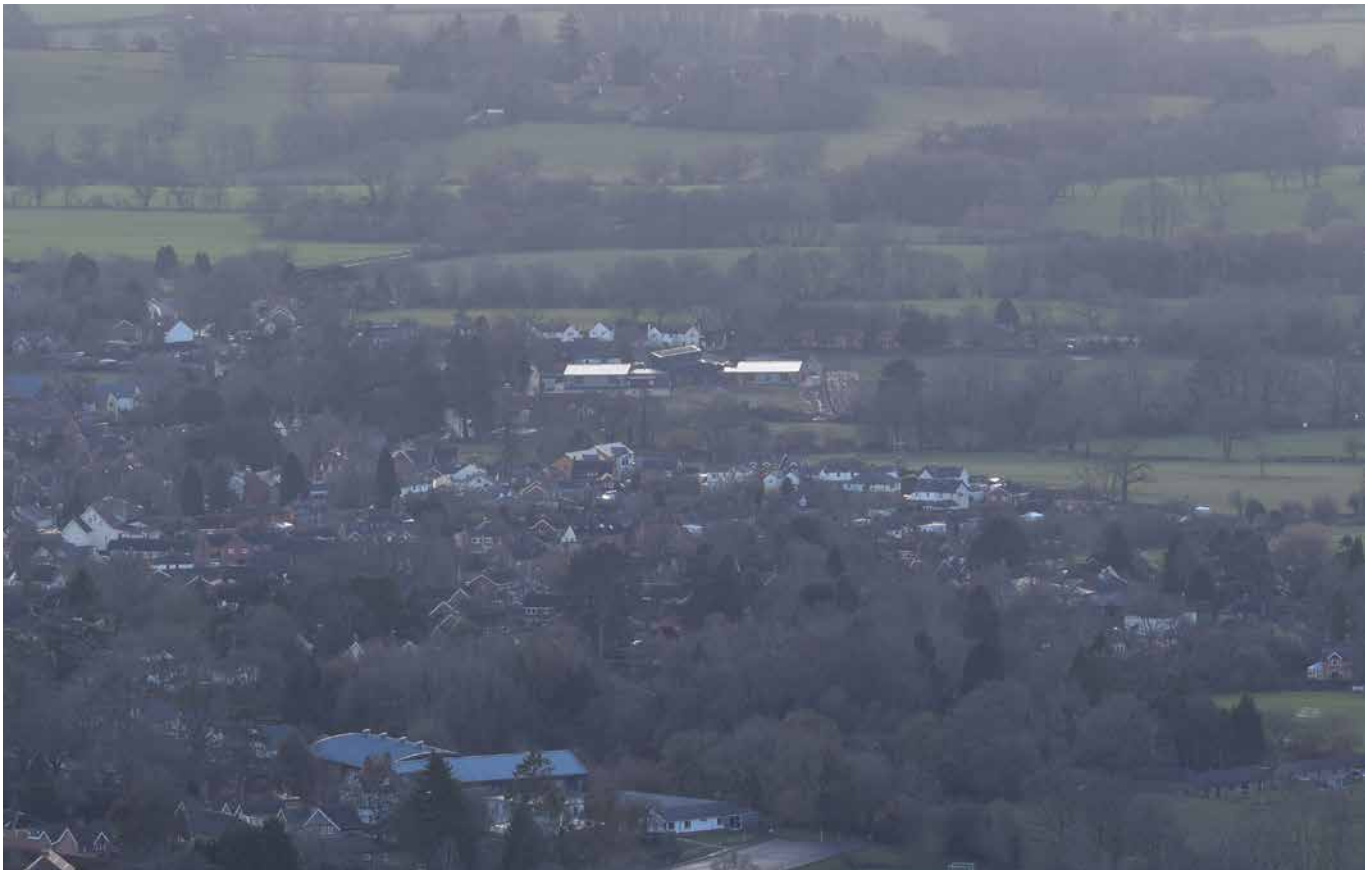
Figure 12 Polymer coating on two low roofs (centre of image) gives rise to significant glare
