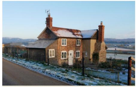
Timber extensions to the west and east of the original cottage are discrete and modestly proportioned. New external chimney stack follows traditional design, with stone reused from original dwelling and new bricks selected to match the original.
