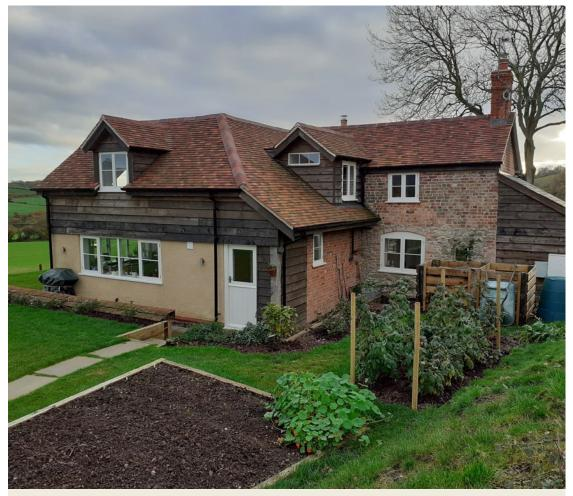
Recessive colours applied to the larch cladding are sympathetic to the original brickwork façades, and visually 'push back' the extensions. Textured render in a warm colour brings out the warmth and tactile nature of the original brick and masonry. Careful brick and mortar selection for new masonry fits well with the original.
