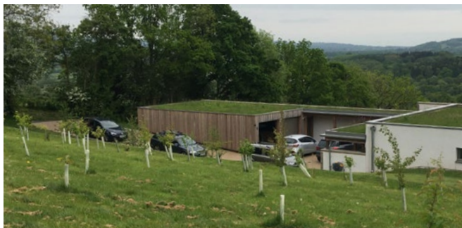
The visual complexity of entranceways, garages and car parking is hidden from view behind the extended curtain wall, presenting a simple continuous façade to the main viewpoint.
