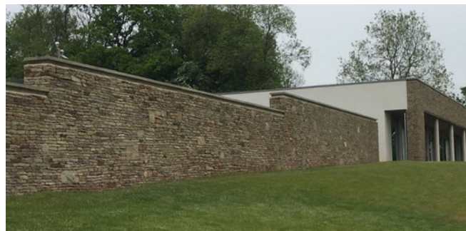
The use of traditional stone to the most visible elevations is contrasted with the cool contemporary precision of the rendered hillside elevations.
