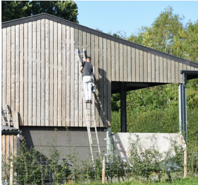
Post-construction treatment to the timber cladding with a darker semi-transparent wood stain reduces the tonal contrast between the concrete planks and the timber. This reduces the overall perception of height.
