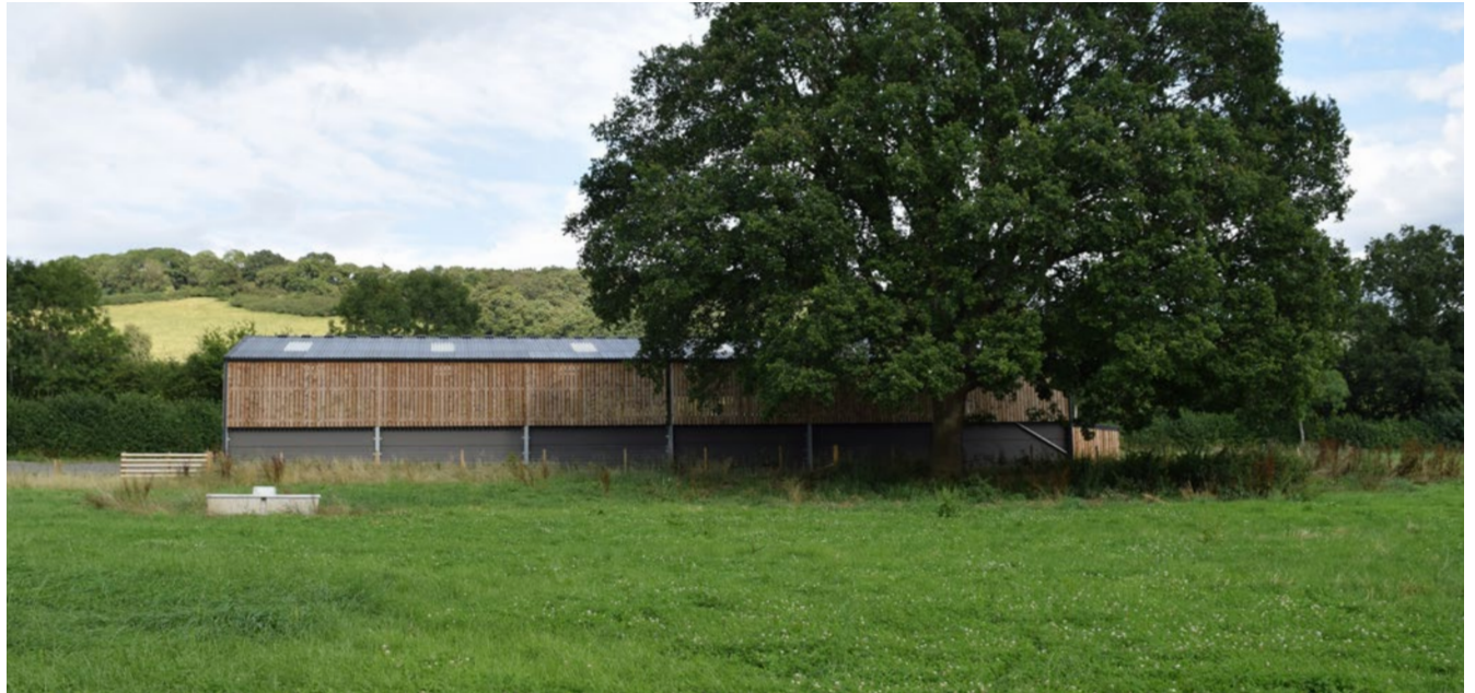
Treating the concrete panels to match the tonal value of the ground it sits on, sets the building back down on the earth and reduces the overall perception of height. The contrast in materials puts a 'waistline' on the building which diminishes its apparent scale. The fibre cement roof is dark grey and non-reflective, unlike sheet metal roofs. This helps the barn to recede within views, especially when seen from the hills above.
