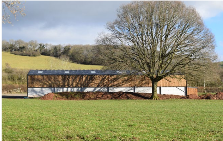
The untreated concrete plank panels visually lift the barn off the ground and the extreme tonal contrast between earth and concrete draws attention to the whole structure.
