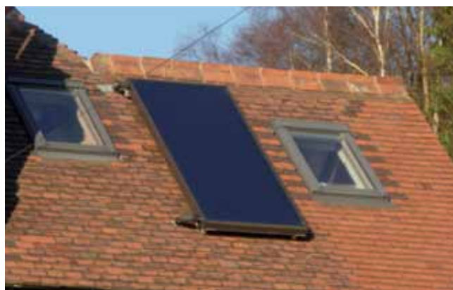
Dark non-reflective solar water heater
