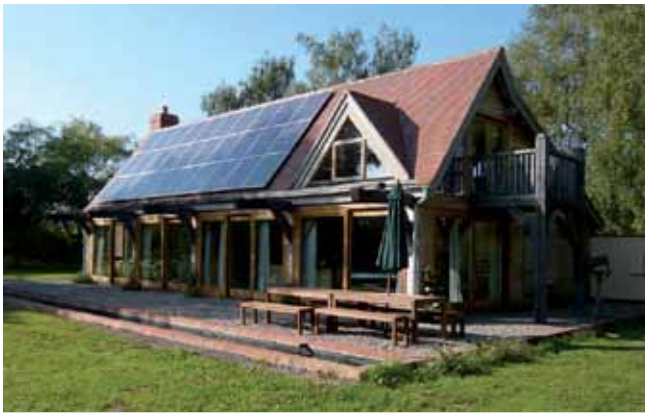
The impact of large areas of glazing is reduced by a timber canopy and by anti-reflection glass that is broken up by timber
