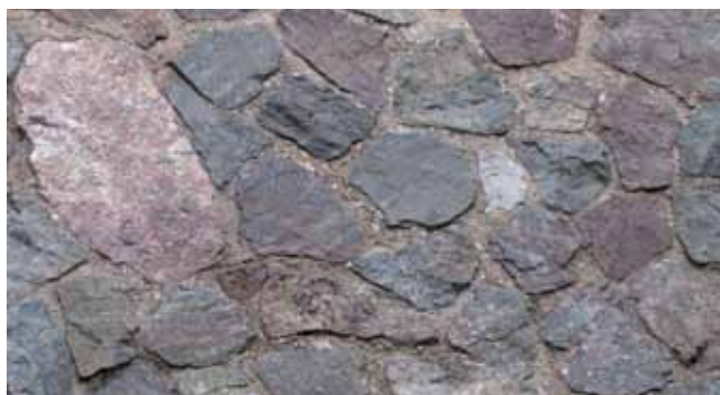
Malvern stone with soft mortar
