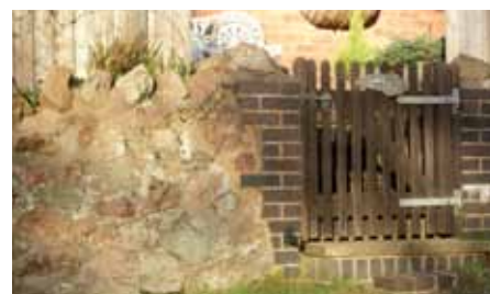
Malvern stone wall ending in blue brick
