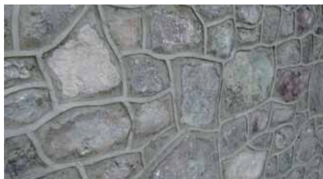
Snake/ribbon pointing on Malvern stone wall
