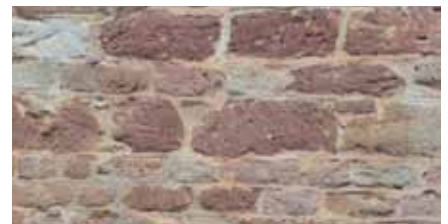
Coursed rubble sandstone stone wall
