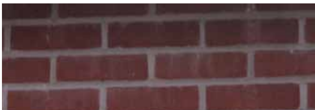
Hard, white mortar is uncharacteristic of the area
