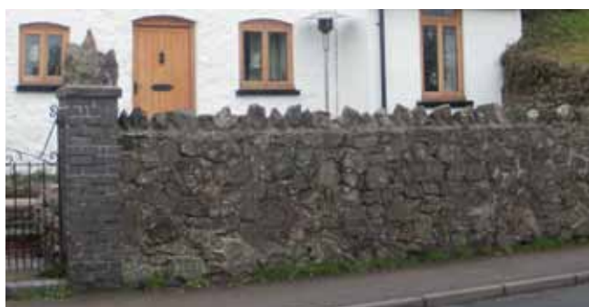
Malvern stone boundary ending in blue brick
