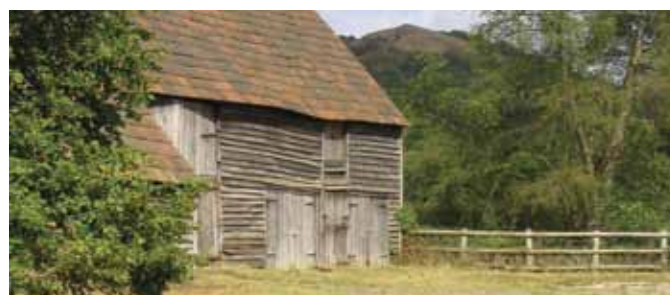
Weatherboarding is a typical feature of many farm buildings
