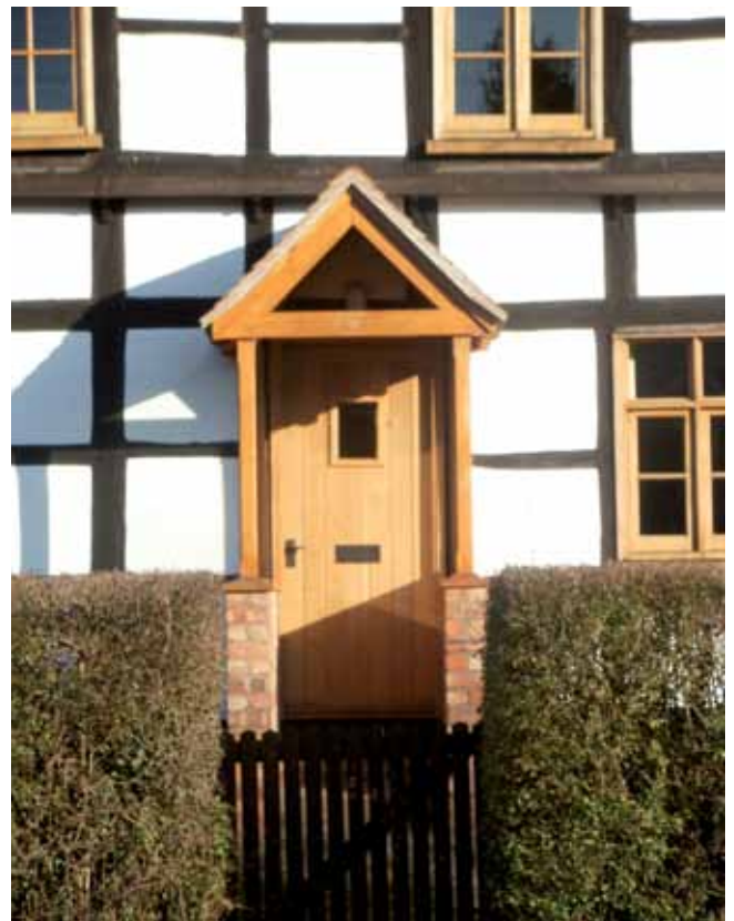
This new timber door respects the building's scale, being no larger than the original opening. The porch respects scale and complements the door
