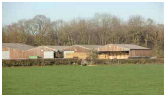
Portal-framed sheds such as these are vital for the modern farming industry. Vertical timber boarding complements the trees behind
