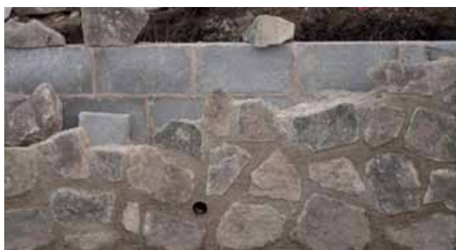
Malvern stone facing a breeze block wall
